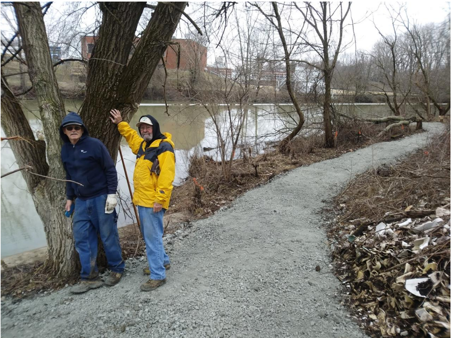
Finished Portage Trail at Low Head Dam (Waterworks Dam)
